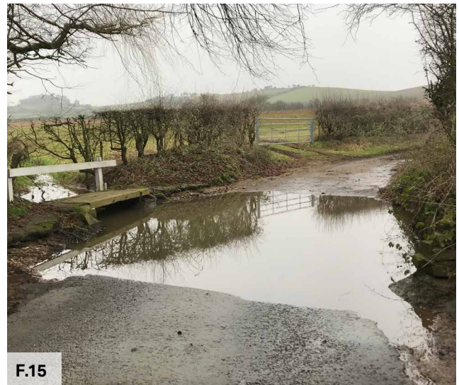
Figure 15: Flooding in Ings Lane, Belchford
